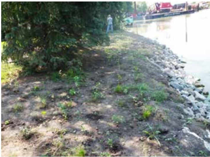
Stream bank erosion is mitigated on Sawyer Creek with riprap and native plantings using funds from the Utica settlement. Photo courtesy of Winnebago Land and Water Conservation Department.
